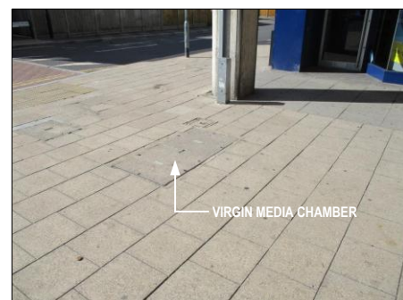
PHOTOGRAPH 3 EXISTING VIRGIN MEDIA CHAMBER IN FOOTWAY AT SOUTH EAST CORNER OF BUILDING
