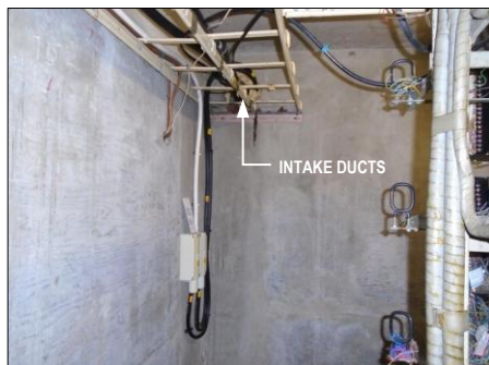
PHOTOGRAPH 7 EXISTING BT DUCT ENTRIES IN BASEMENT ON EASTERN ELEVATION OF BUILDING IN BT FRAME ROOM
