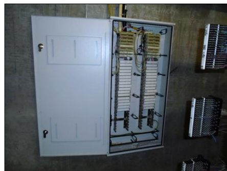
PHOTOGRAPH 8 EXISTING BT COPPER DISTRIBUTION POINT ON WALL IN BT FRAME ROOM IN BASEMENT
