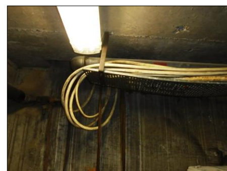
PHOTOGRAPH 12 EXISTING BT COPPER AND FIBRE SERVICES ACCESSING RISER IN BASEMENT PLANT ROOM
