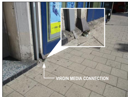
PHOTOGRAPH 5 EXISTING VIRGIN MEDIA CONNECTION TO BUILDING ON GRAFTON ROAD AT FOOTWAY LEVEL
