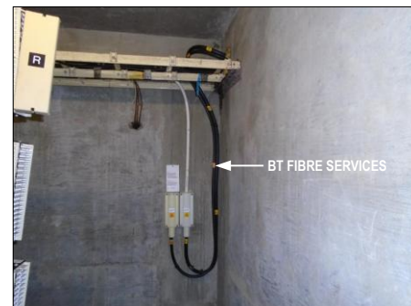
PHOTOGRAPH 9 EXISTING INCOMING / OUTGOING FIBRE SERVICES AND GAS SEALS ADJACENT TO DUCT INTAKES IN BT FRAME ROOM
