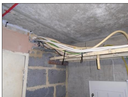
PHOTOGRAPH 10 EXISTING BT CABLING EXITING FRAME ROOM ON HIGH LEVEL CONTAINMENT TO BASEMENT CORRIDOR
