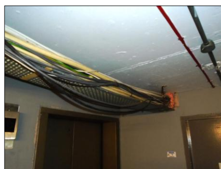
PHOTOGRAPH 11 EXISTING BT COPPER AND FIBRE SERVICES ON HIGH LEVEL CONTAINMENT IN BASEMENT CORRIDOR TO RISER
