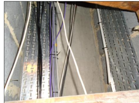
PHOTOGRAPH 15 TYPICAL VIEW OF RISER ON UPPER FLOOR OF VACANT SUITE INDICATING SERVICES AND AVAILABLE SPACE
